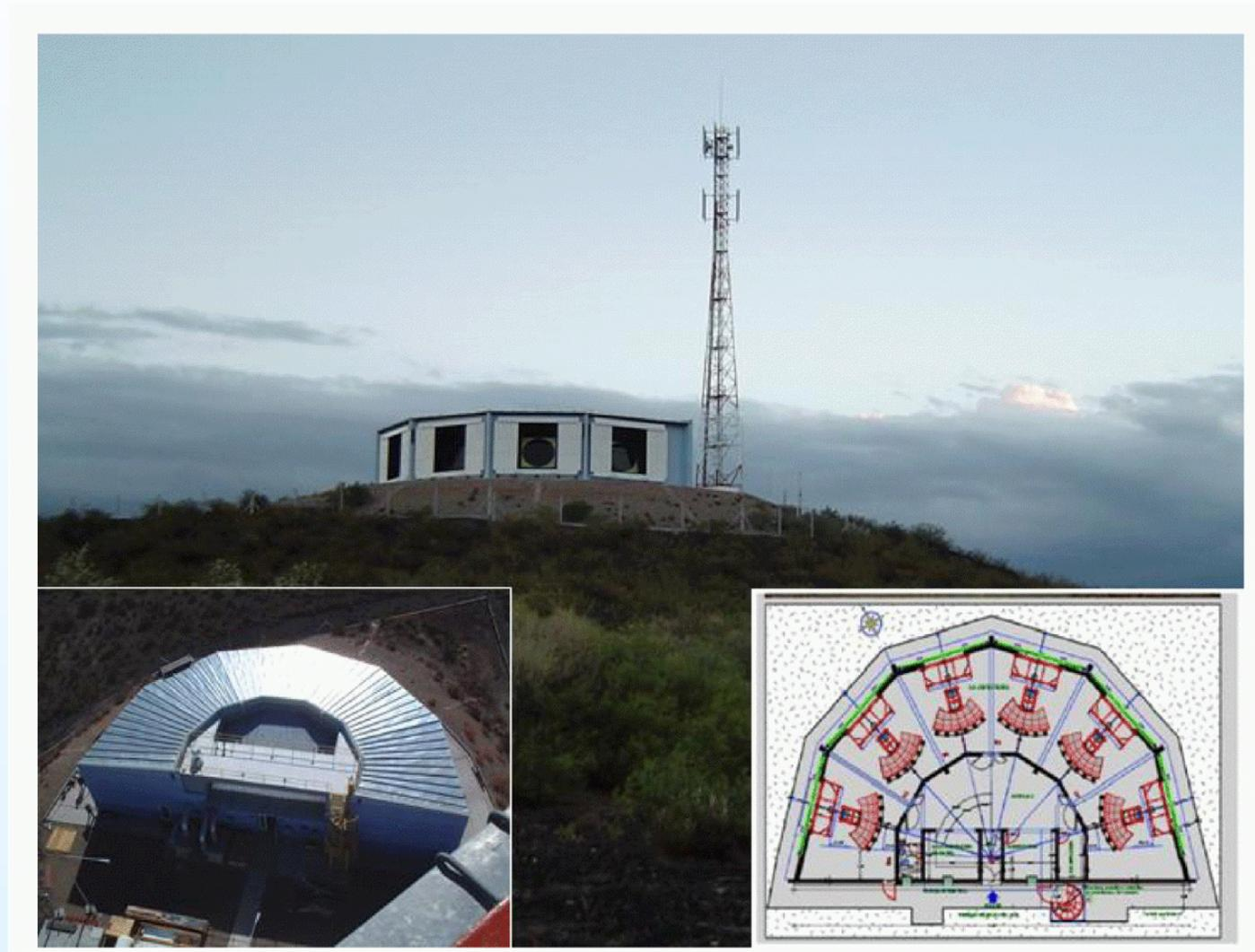
One of four Fluorescence Detectors. Each FD includes 6 telescopes.
